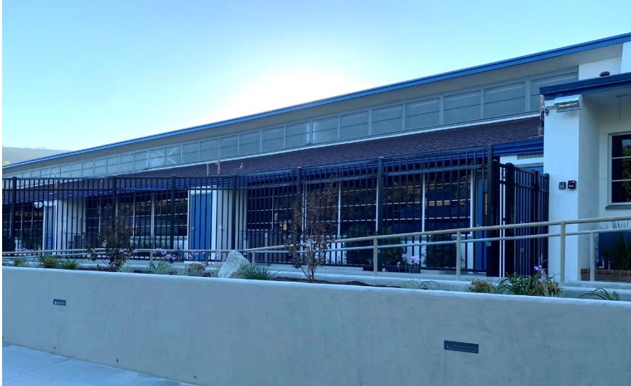
Front Security Fencing
